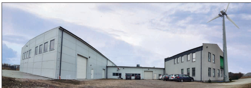
FIGURE 2 – The headquarters of the technology company MMB Drives has its own power sources in the form of a wind farm, photovoltaic panels, and heat pump.
